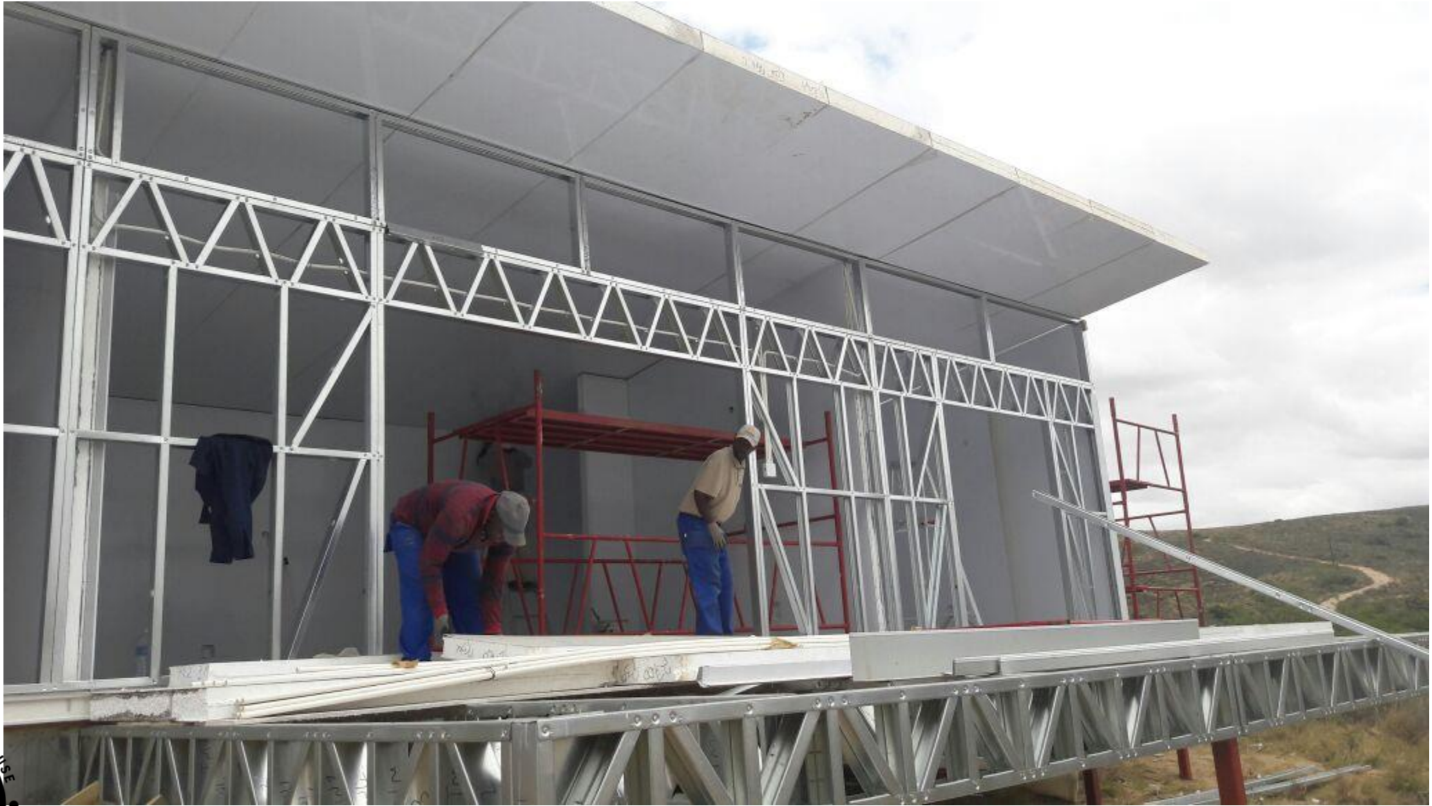
Hybridisation Thermal Panels and Lightweight Steel Frame Construction
